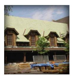
After finding several 90-year-old clay roof tiles in the field house attic, **Knickerbocker Roofing** contacted the original tile manufacturer, Ludowici Roof Tile, and asked them to replicate the tile with one of their modern products. Ludowici matched the style to their current large-size Classic XL tile product, and then custom manufactured the tiles in a shade of green that matches the original color.
