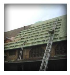
The original 1914 Pulaski Park Field House had a green Ludowici Roof Tile roof system on the 49,100-square-foot (4561-m²) facility, which has a 12-in-12 (45-degree) slope. A Spanish clay tile roof system was installed on the 6,000-square-foot (557-m²) veranda on the south side of the building, which has a 3-in-12 (14-degree) slope. Both roof systems had a 1 1/8-inch- (29-mm-) thick tongue-and-groove wood deck substrate.
