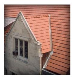
Next, one layer of 5/8-inch- (15.6-mm-) thick Dens-Deck® and one layer of 3/4-inch- (18.8-mm-) thick plywood were mechanically attached. Then, one ply of self-adhering Grace Ice and Water Shield was installed followed by two plies of No. 30 asphalt felt that was secured by 1-inch (25-mm) diameter head disk nails. Finally, interlocking Ludowici Classic<sup>TM</sup> Tiles in Clay Red were laid in place.
